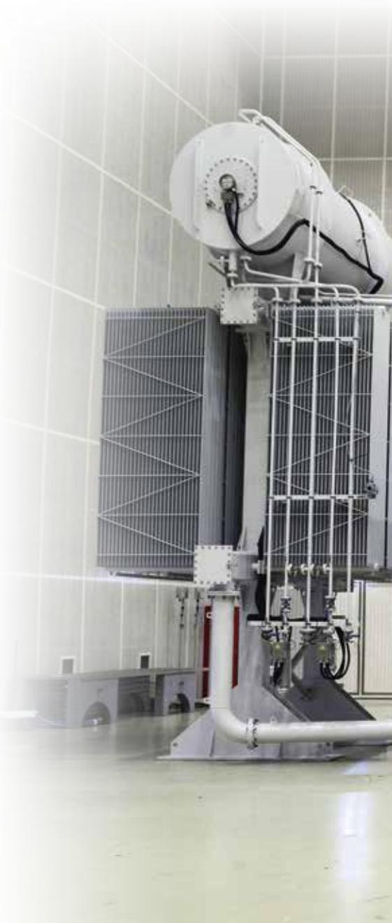
densities like in this transformer, these are not a major issue. The tricky part is to install the noise dampers with the insulation panels. This requires precise planning and skilled handwork.
